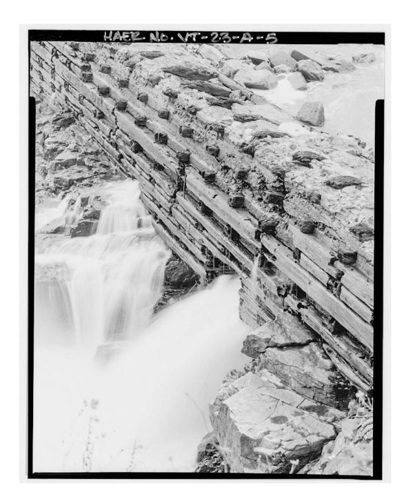
This dam was located upstream from the Salmon Hole on the Winooski River. Built in 1876, it is a notable example of a timber-crib dam and one of the first to use concrete as a crib fill. The dam was an essential part of the mill system, providing the hydroelectric energy necessary to produce goods.
